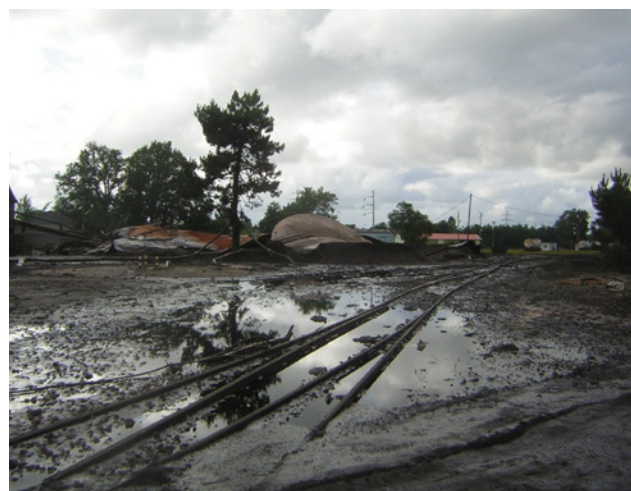
Photographs of the tank taken before and after the accident - Source: DREAL Aquitaine (Environmental Agency)
